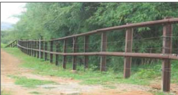
**Figure 5.** Railway line barrier with integrated electric fencing.
