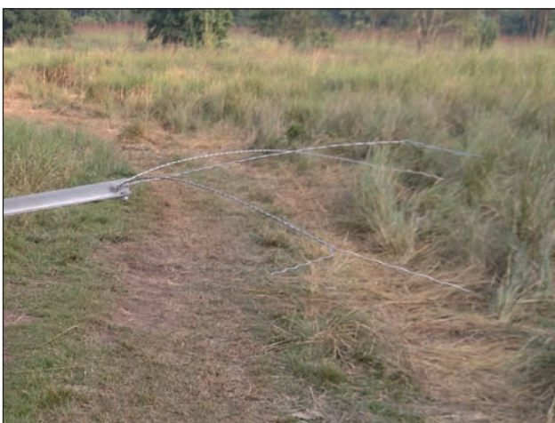
Figure 5. Electrified ‘whiskers’ that extend from the tip of the brace protect the brace from being targeted by elephant.
