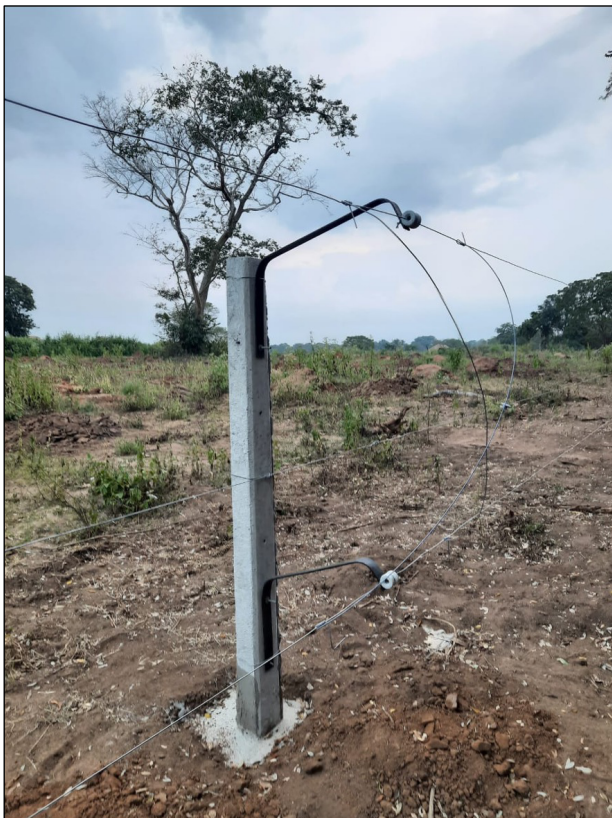
Figure 1. Modified concrete post.
